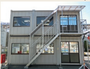
5 Risk awareness equipment Employees are trained here to enhance their risk awareness and develop their ability to detect potential hazards in their day-to-day work.
