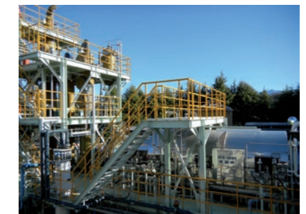
Detoxification equipment for greenhouse gas
