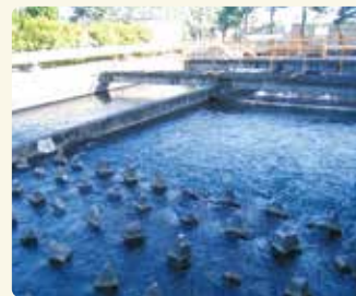
Discharged water (cleaned at the plant)
