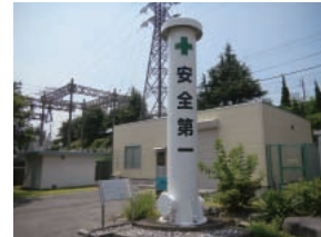
The safety first tower
